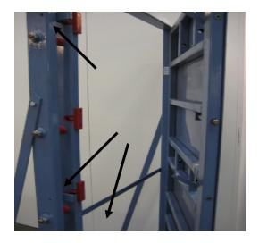
Before mounting the door should be looked at all 4 places. 3 places with breakable pins and one place with the fixed locking point.
